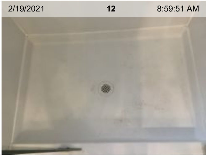
Shower/Fixture | Base of Shower
