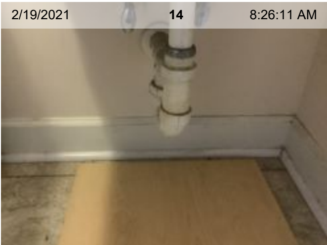
Cabinet Under Sink
