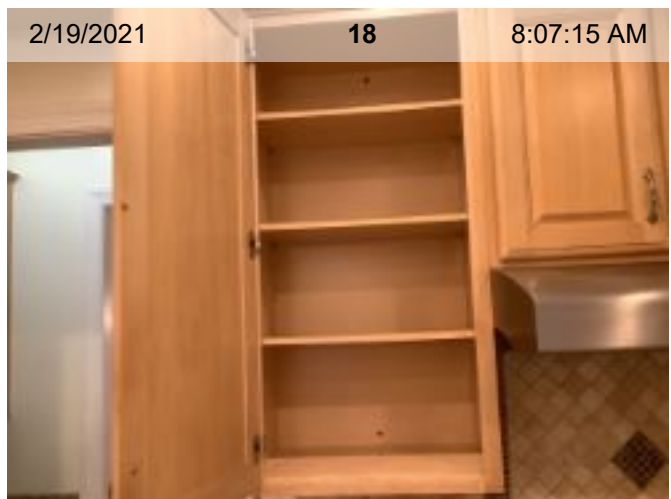
2/19/2021 18 8:07:15 AM Upper Cabinets | Interior
