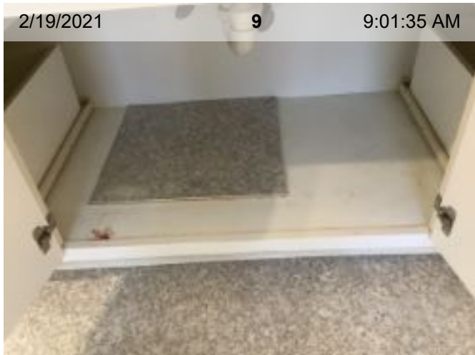
Cabinet Under Sink
