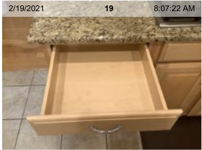
Lower Cabinets | Interior
