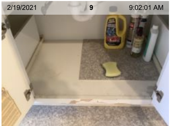
Cabinet Under Sink
