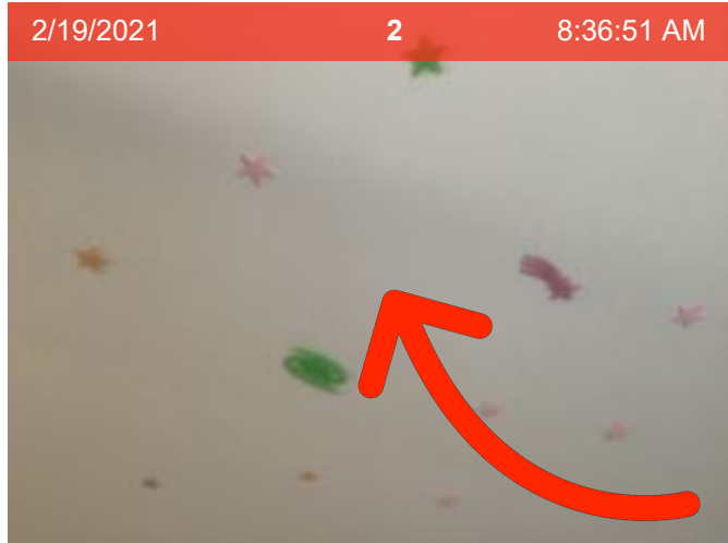
Ceiling | Stickers on ceiling.
