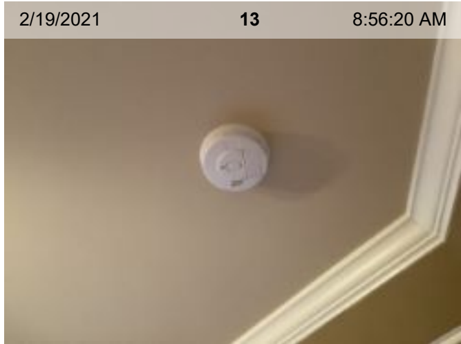
Wired Smoke Alarm (mfd 1/2015) | Smoke test: Passed | Alarm in place (on ceiling or wall)
