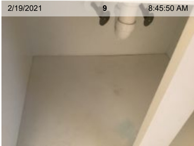
Cabinet Under Sink
