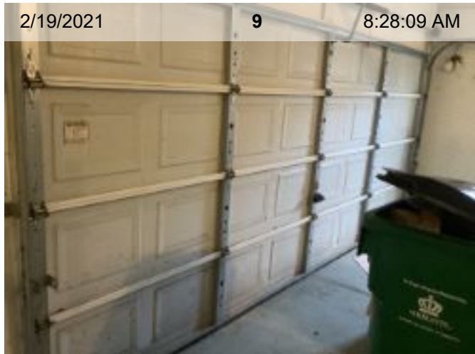
Garage Door Interior
