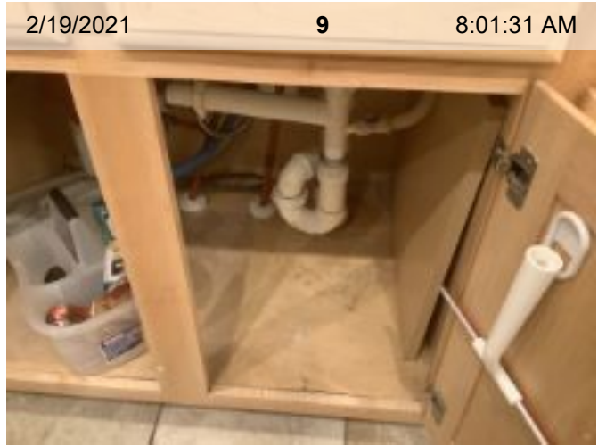
Cabinet Under Sink
