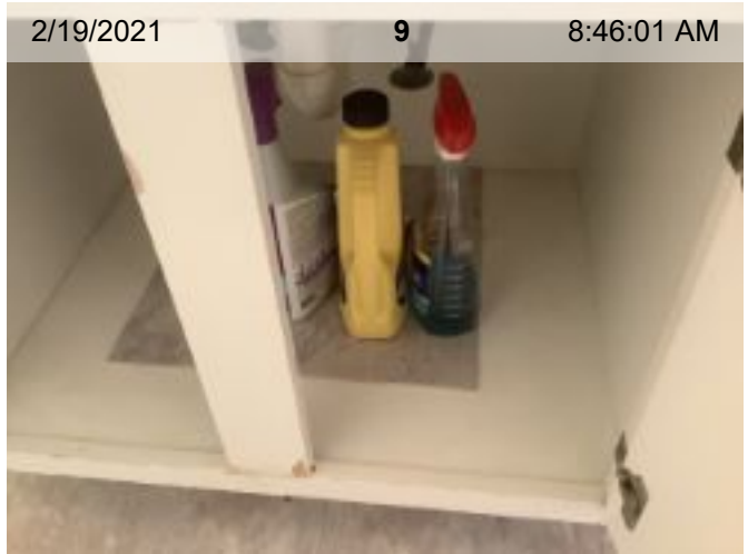
Cabinet Under Sink
