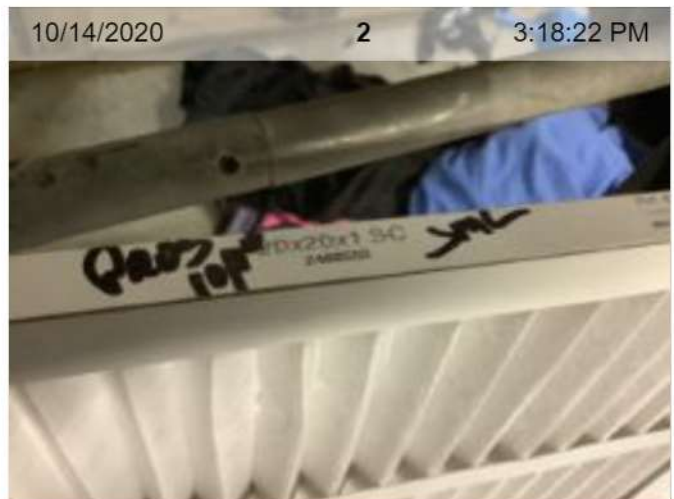
20 x 20 x 1 Air Filter Installed | Close-up of size/initials/date
