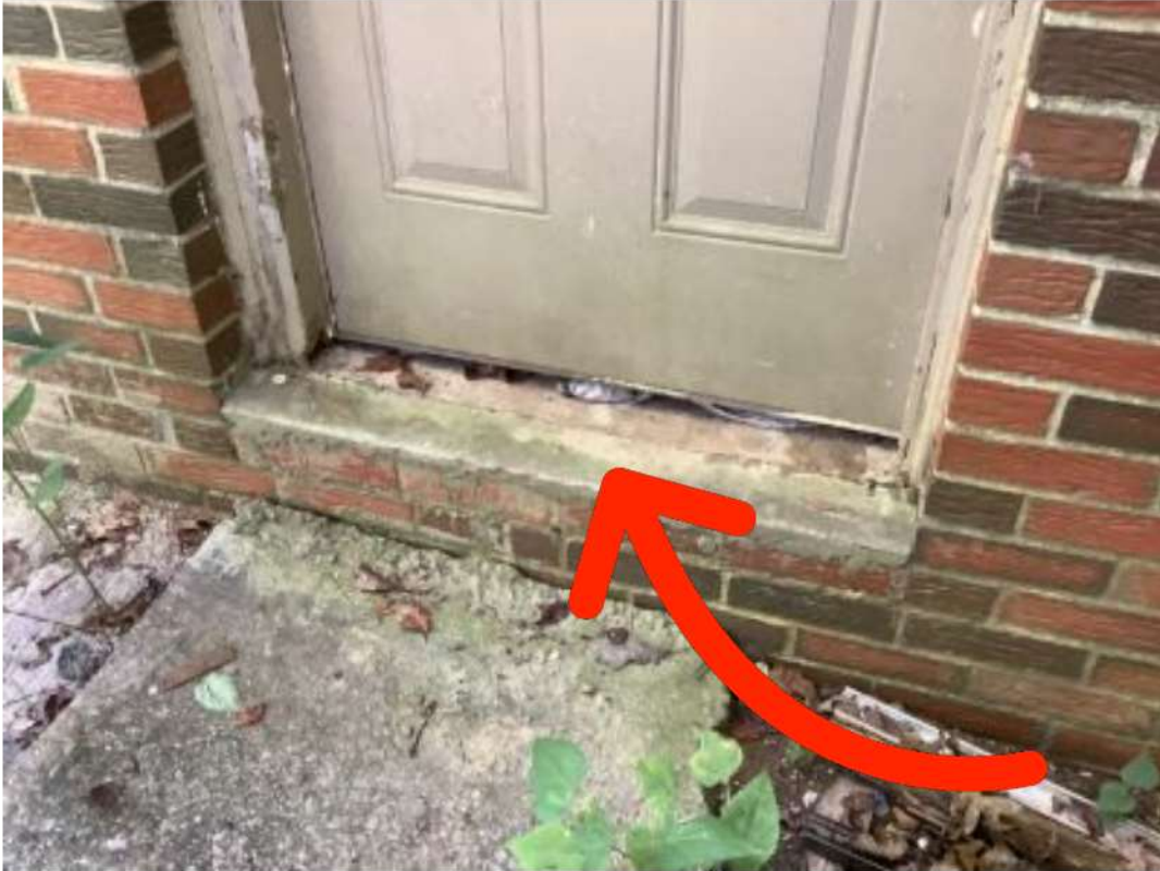
Rear Exterior Rear Door Gap under back door
