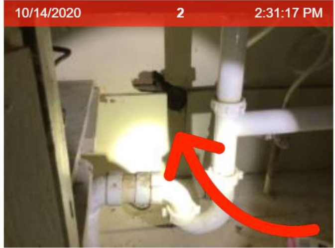
Cabinet Under Sink
