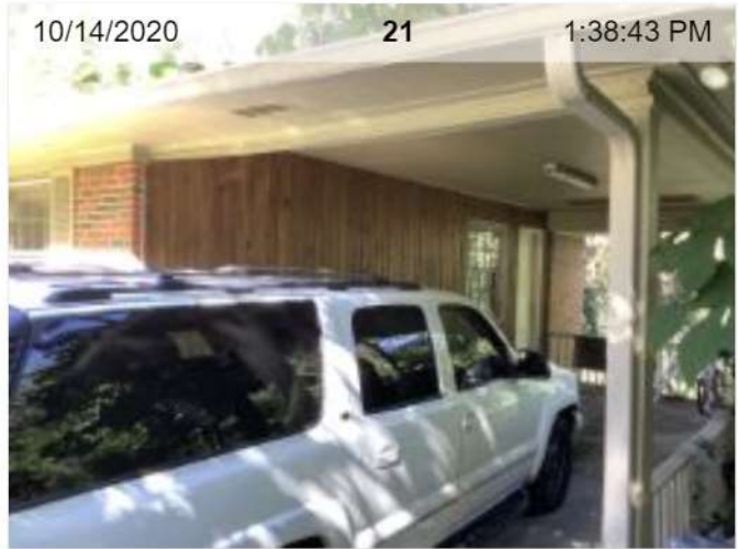
Walls/Siding/Trim | Left, Front, and Right Sides
