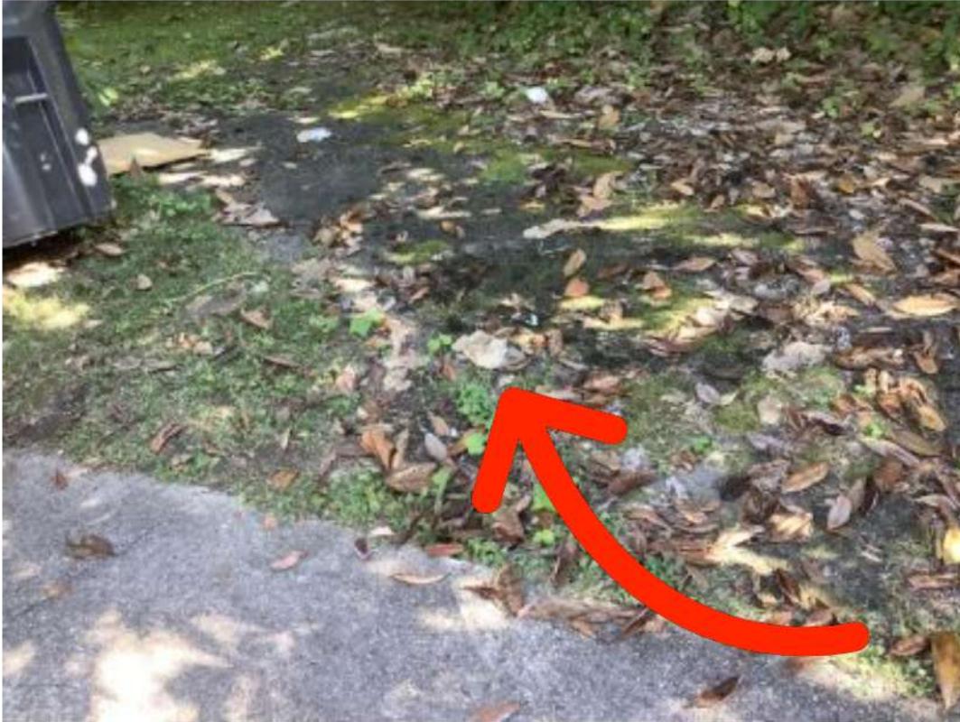
Front Exterior Drainage Issues Right side of house
