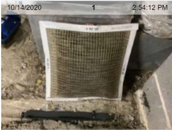
20 x 20 x 1 Air Filter Removed | Front
