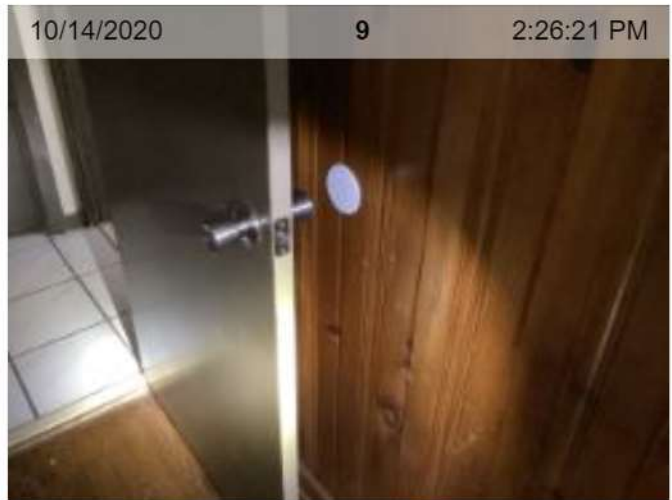
Door Stop Installed
