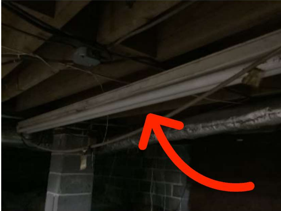
Basement Light Fixtures Does not turn on
