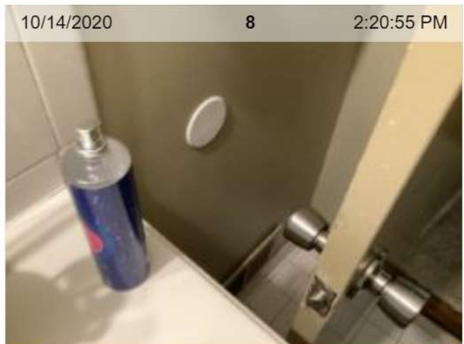
Door Stop Installed
