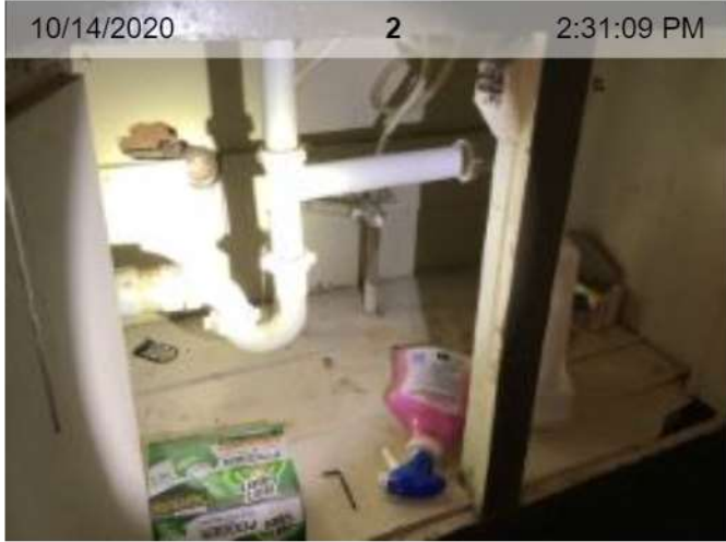
Cabinet Under Sink
