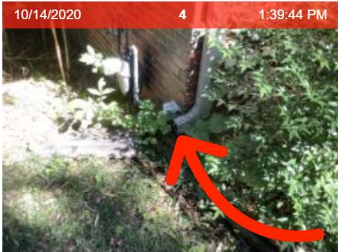
Downspout/Splash Blocks | Splash guard moved
